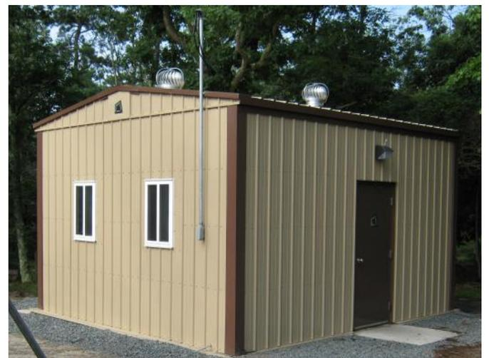
Building with Wind Driven Roof Ventilators
