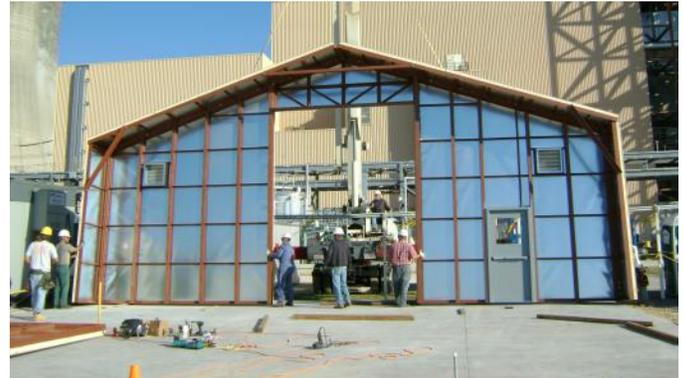
Endwall Being Set with Factory Installed Personnel Door,
