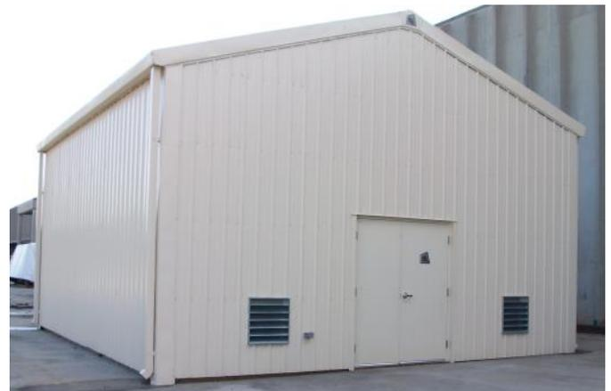
Building with Factory Installed Intake Louvers
