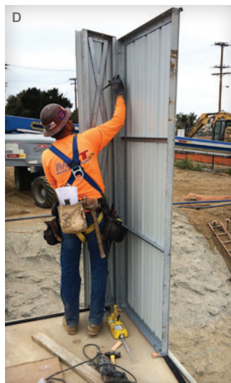
A&B: Installing wall panels with boom lift C: Finished tide gate enclosure D: Bolting together wall panels from the inside E: Factory installed door panel arrives
