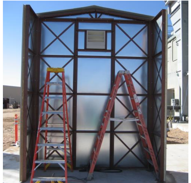
Additional panels create the first complete end-wall. A gable closure panel with factory attached trim creates the start of the gable roof shape.
