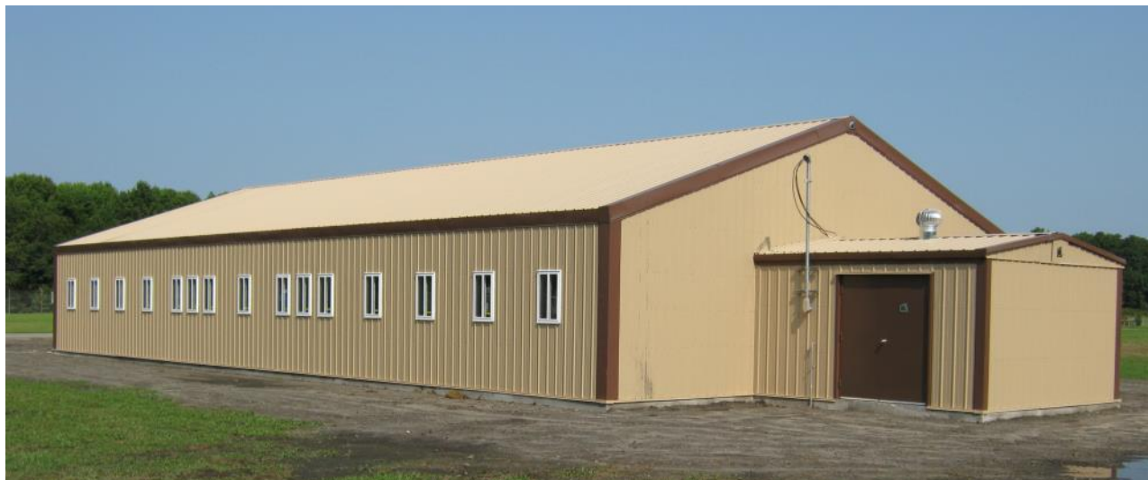
This 42' wide x 81' long classroom building was installed using troop labor without prior experience during a two week training deployment at Fort Dix in New Jersey.
