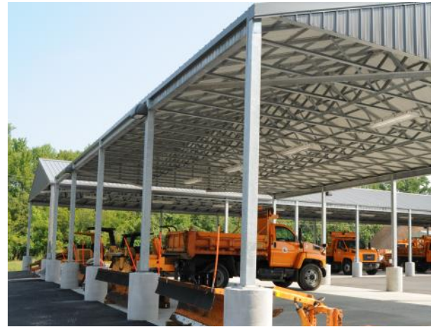
Canopy at County of Henrico, VA Maintenance Yard
