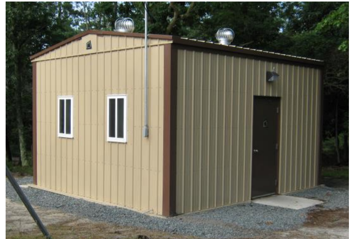
Building with 2' Wide x 3' High Sliding Vinyl Windows Factory Installed in Two Wall Panels
