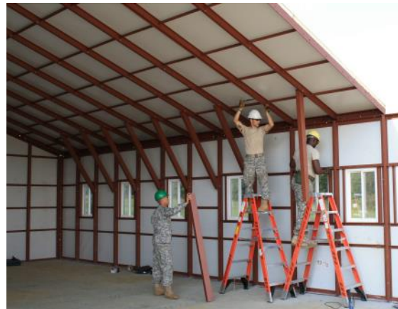
Knee and ridge braces are installed as wall and roof panel sections are set in place.
