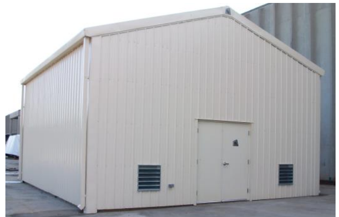
Building with Factory Installed Intake Louvers
