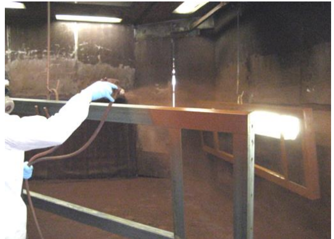
The Standard Red Primer Being Applied
