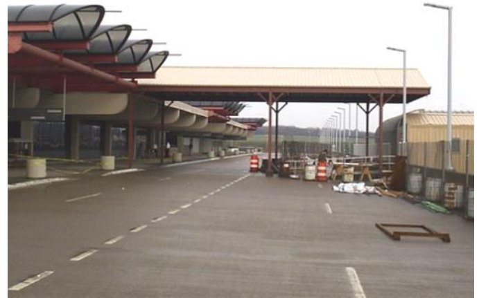
Passenger Walkway Cover at Pittsburgh International Airport
