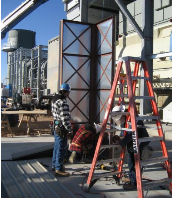
Two wall panels and a corner erection angle make the first corner of the building.
