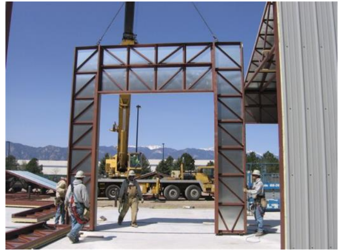
A Factory Reinforced Equipment Door Opening in the Building’s Sidewall Being Lifted Into Place
