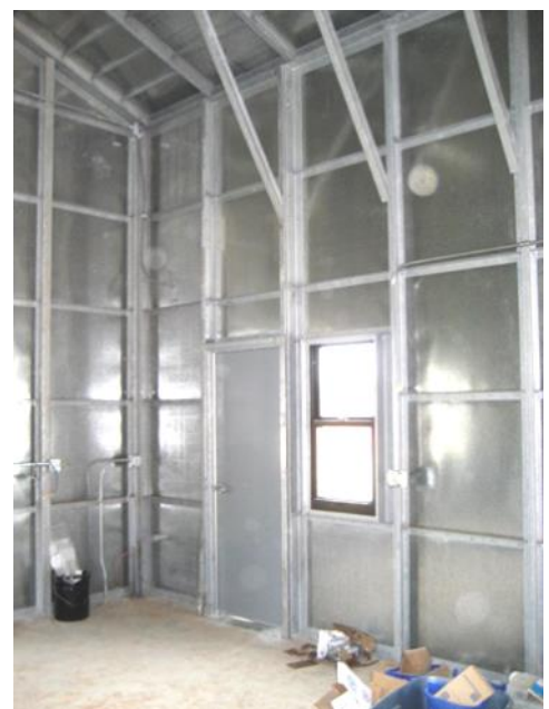
A Building's Interior with Hot-Dip Galvanized Frames in the Gulf Coast Region
