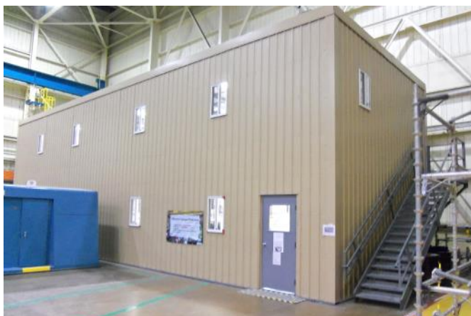
2-Story Office and Break Room Building
