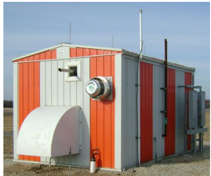
Factory Installed Framing for Ventilation Penetrations
