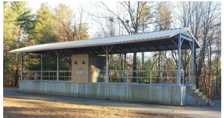
Water Point Canopy at Fort Devens, MA
