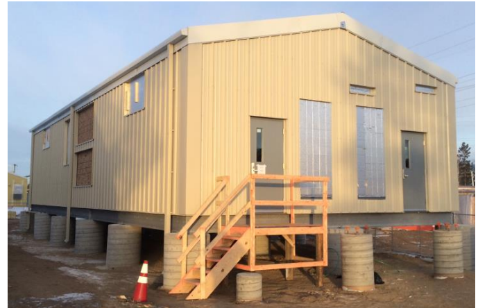
MCC Building with Factory Framed Cable Tray and HVAC Penetrations
