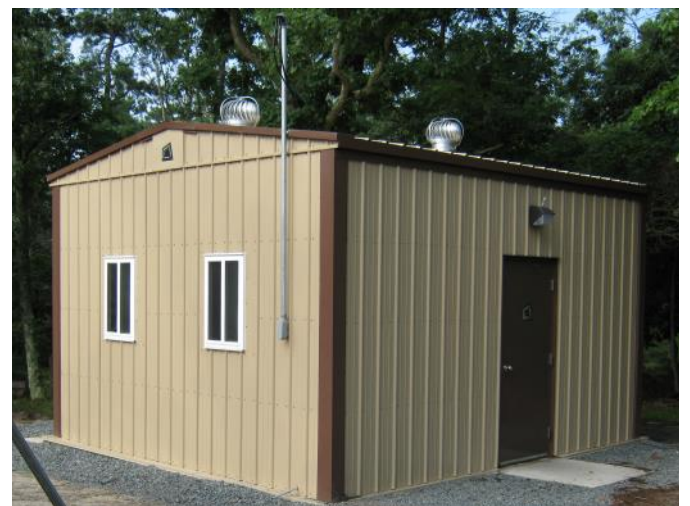
Building with Wind Driven Roof Ventilators
