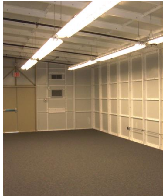
Painted Steel Liner
