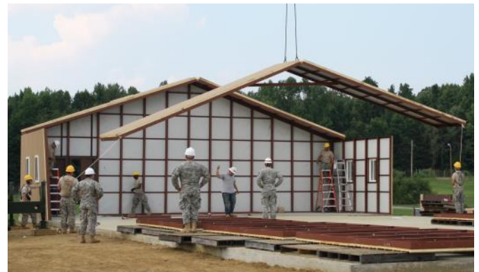
6' roof sections are assembled on the ground and lifted into place by the crane.
