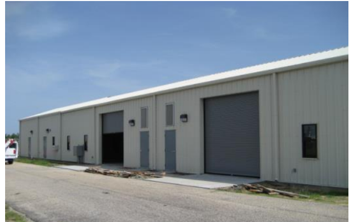
Building with Hurricane Rated Doors & Windows
