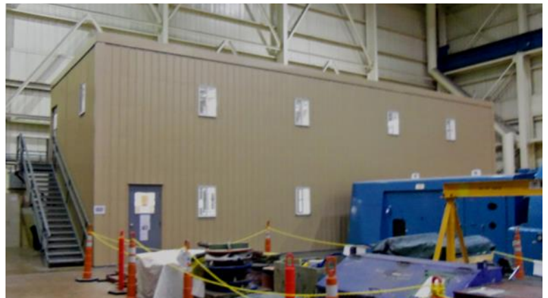
Two-Story Office & Break Room Located on the Turbine Deck at a Power Plant
