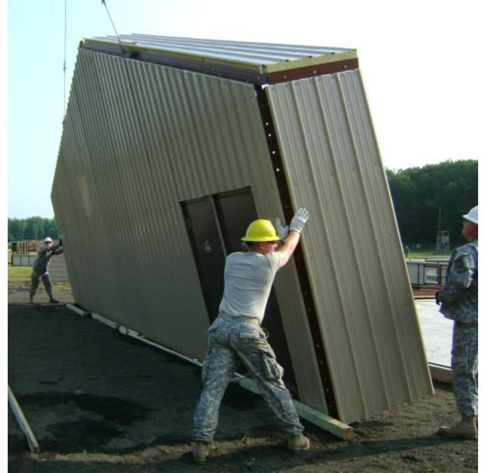
The endwall and 3' of sidewall and roof are lifted into place with a crane.
