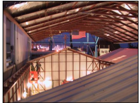
Roof Section Being Lifted From Building for Turbine Access during Power Plant Outage
