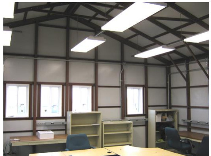
Building with Factory Installed Windows
