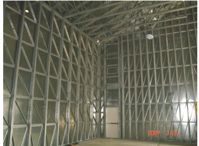
Interior of Building Rated for 180 MPH Wind Load in Okinawa, Japan with Hot-Dip Galvanized Steel Framing
