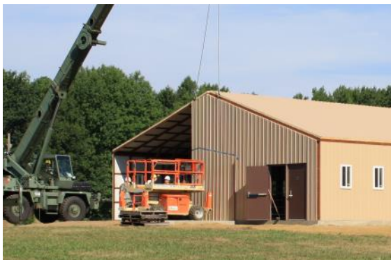
The final endwall is added. Trim and flashing are installed to complete the building.
