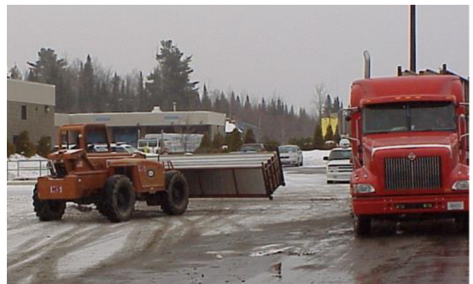
Rack of Panels Being Moved by Telehandler
