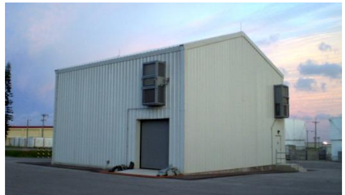
Building Rated for 180 MPH Wind in Okinawa, Japan
