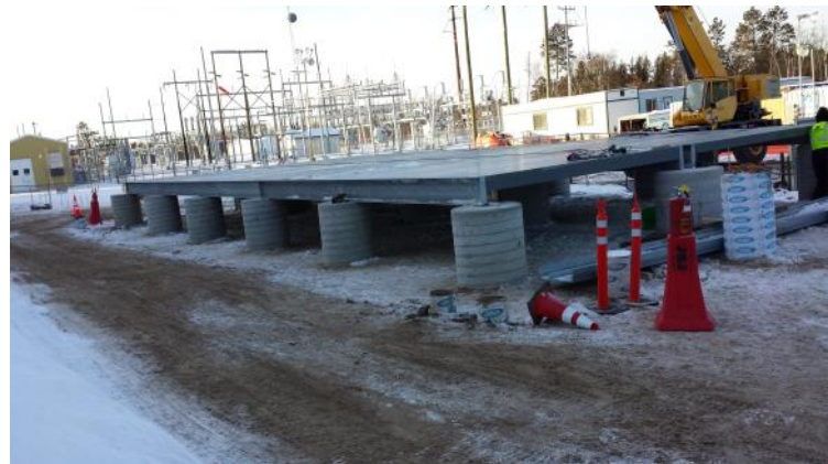
Floor System Assembled on Pier Supports
