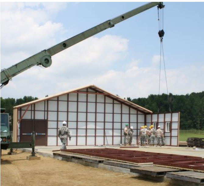
Sections of sidewall panels are sub-assembled and lifted into place with the crane.
