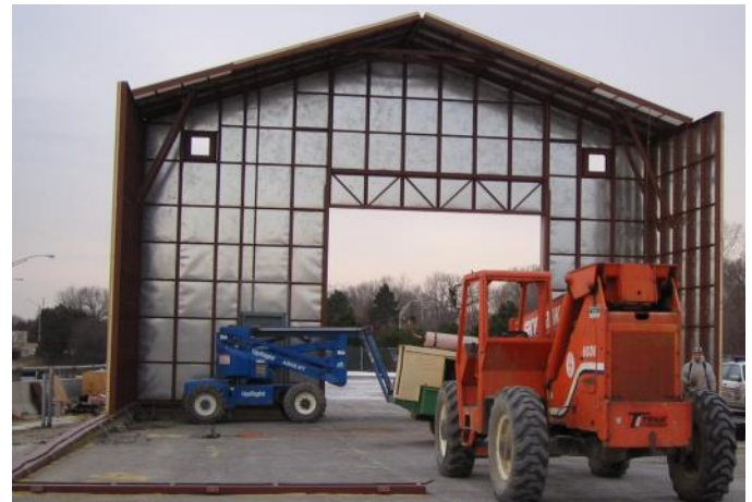
Building Installs on Base Channel Similar to Installation on New Concrete
