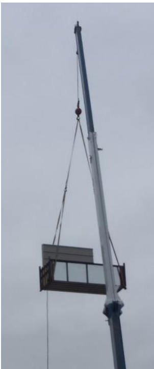
Panel Racks Being Moved with Slings by Overhead Crane
