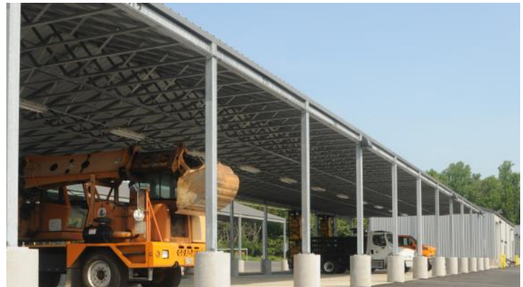
Interior of Building Rated for 180 MPH Wind Load in Okinawa, Japan with Hot-Dip Galvanized Steel Framing
