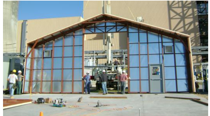
Endwall Being Set with Factory Installed Personnel Door, Louvers and Equipment Door Supports
