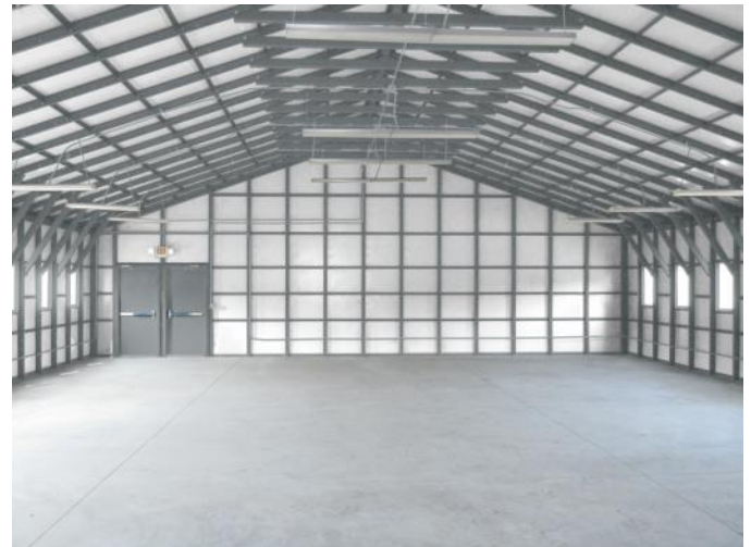
Painted Steel Liner
