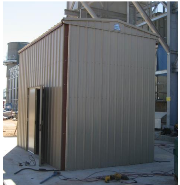
The final endwall installs similar to the first end-wall. Standard trim and flashing is installed to complete the exterior.
