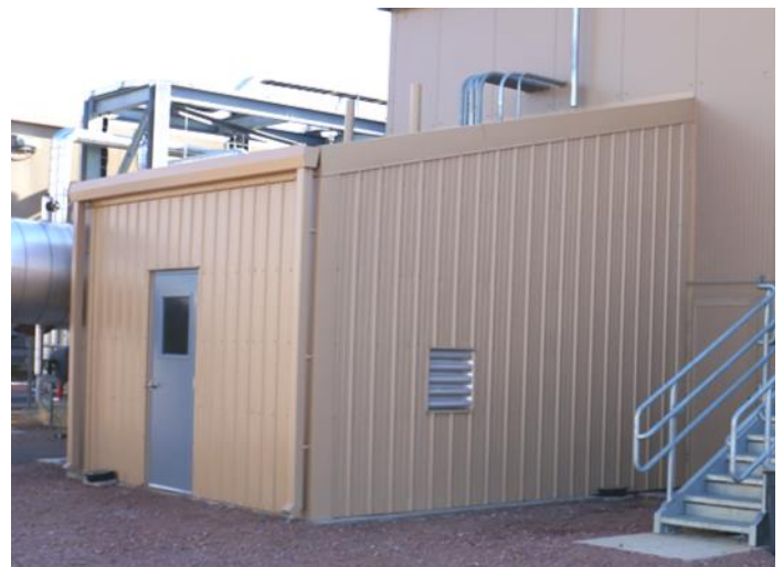
24" x 24" Combination Louver / Damper Factory Installed in Wall Panel
