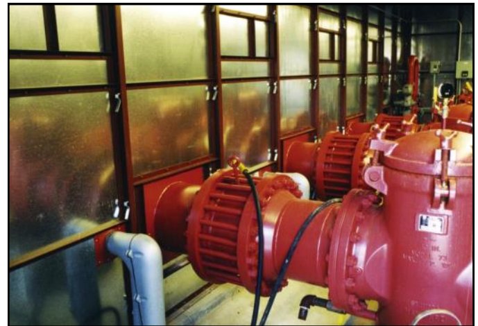
Factory Installed Framing for Pipe Penetrations
