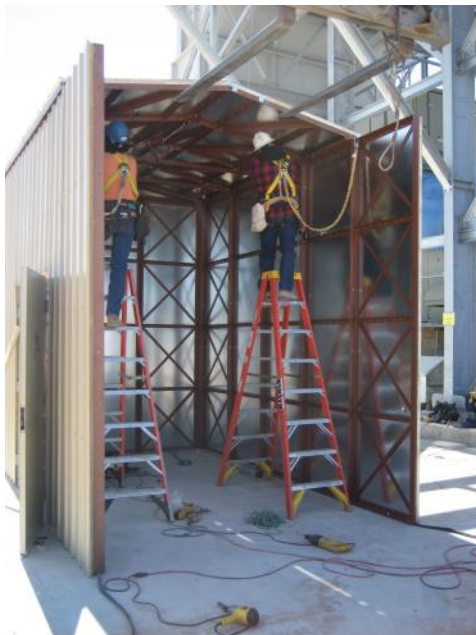
Roof panels are hinged at the ridge. The roof structure is completed with roof trusses comprised of a tension tie and web braces that bolt to the roof panel in the air.
