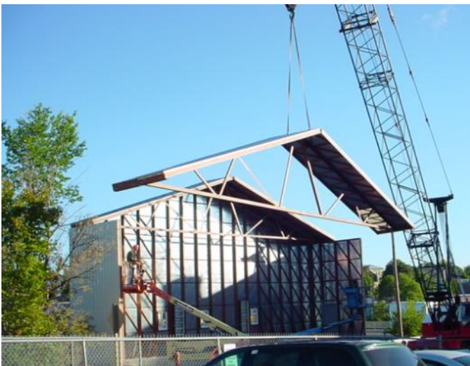
54' Wide Building Using Trussed Roof Structure
