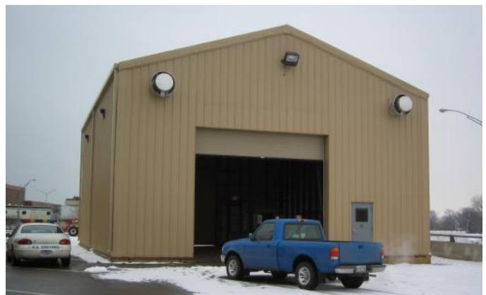
Finished Temporary Vehicle Inspection Enclosure for U.S. Customs and Border Patrol
