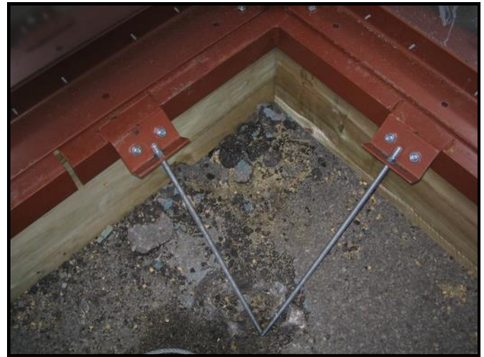
Building Installed on Existing Un-level Asphalt Surface Shimmed with Treated Wood Lumber
