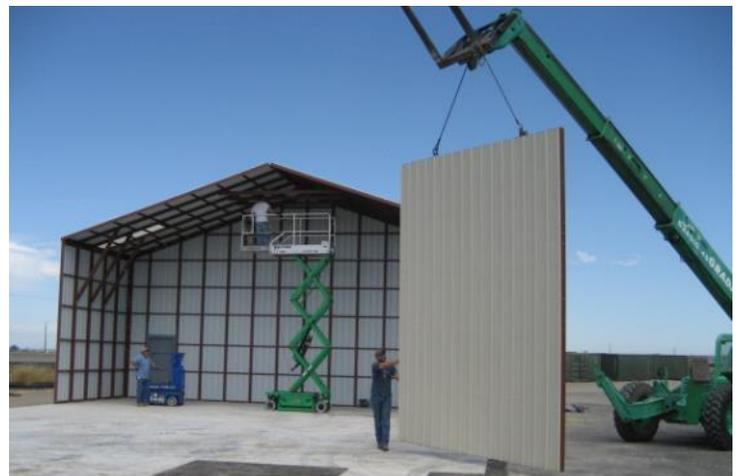
Kelly Klosure’s factory finished panels have an overlapping edge on one panel that corresponds to an underlap edge on the next panel. In the field, as the panels are attached to each other, this overlapping edge creates a weather tight seal without need for stitch screws or sealant.
