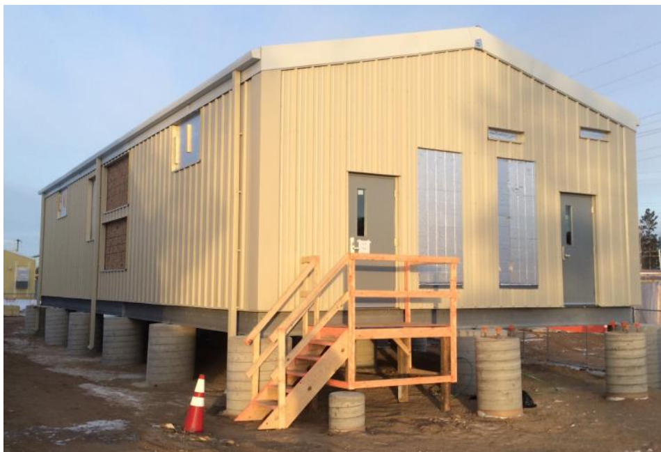
Finished MCC Building on Pier Supports
