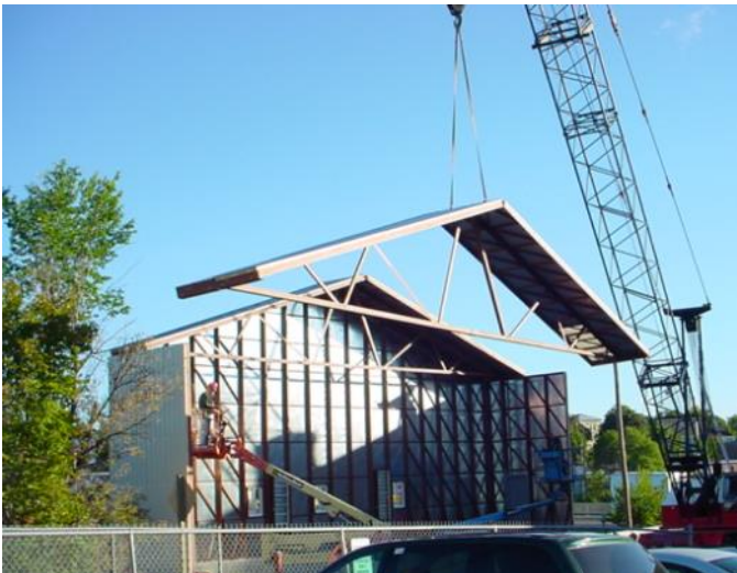
54' Wide Building Using Trussed Roof Structure
