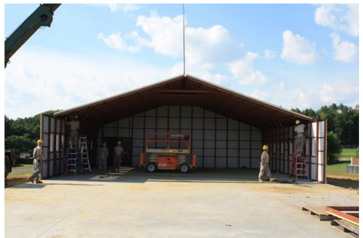
42' Wide Building Using Repetitive Moment Frames (Knee and Ridge Braces)
