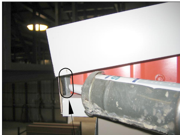
IMPORTANT THIS JOINT NEEDS TO BE CAULKED WELL TO PREVENT WATER FROM ENTERING THE BUILDING.
