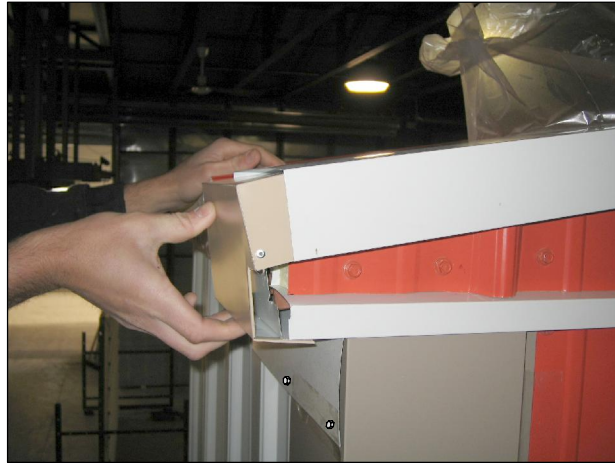
STEP #4 CAULK AROUND THE END CLOSURE CAP AS NECESSARY & INSTALL. NOTE: CLOSURE CAP GOES UNDER RAKE FLASHING & OVER EAVE FLASHING.
