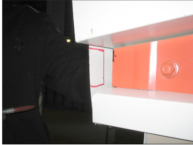
STEP #1 MARK AREA OF EAVE FLASHING THAT IS TO BE REMOVED
