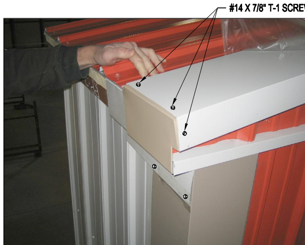
STEP #6 USING SCREWS PROVIDED ATTACH END CLOSURE CAP TO GABLE & EAVE FLASHING.
