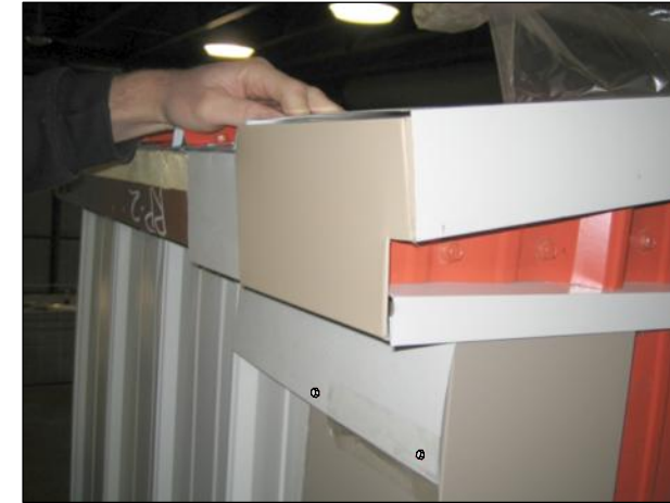
STEP #5 MAKE SURE END CLOSURE CAP HAS BEEN INSTALLED CORRECTLY BEFORE ATTACHING WITH SCREWS.
