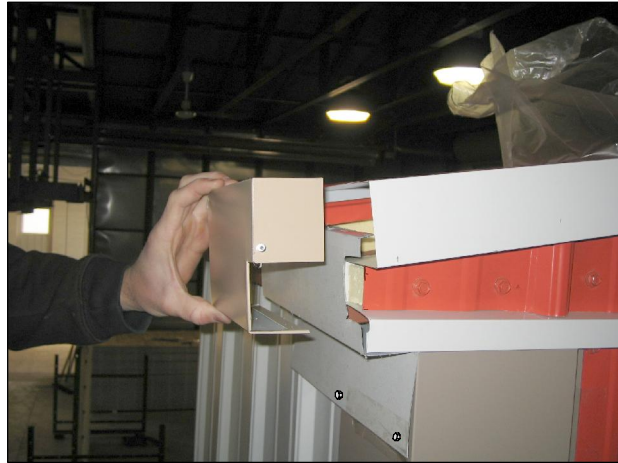
STEP #3 AFTER VERTICAL CORNER CAP & EAVE FLASHING HAS BEEN INSTALLED, INSTALL THE END CLOSURE CAP.
