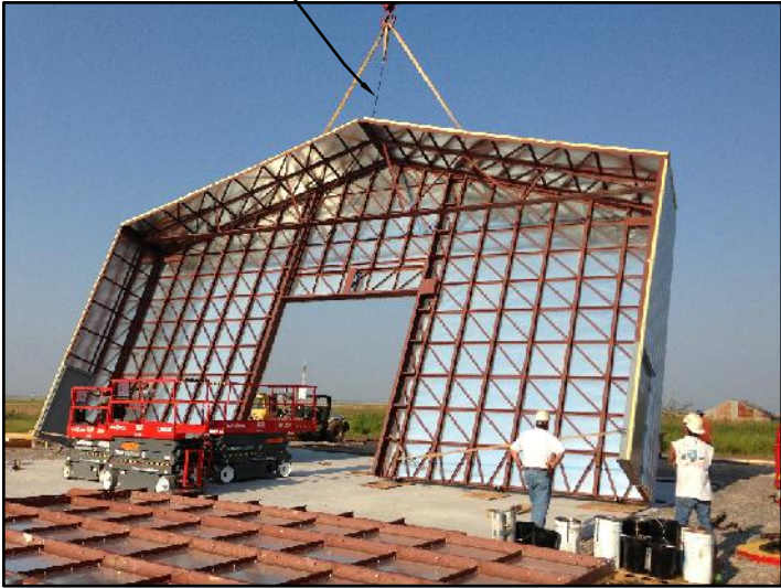
OPTIONALLY USE CHAINFALL RIGGING FOR BETTER CONTROL DURING THE END WALL LIFT.
