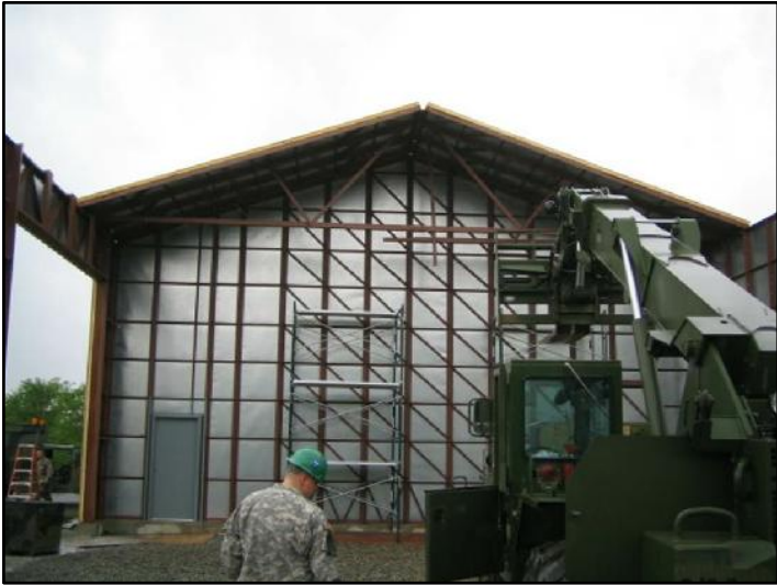
NEXT, INSTALL THE INTERMEDIATE TRUSS & WEB MEMBERS.
