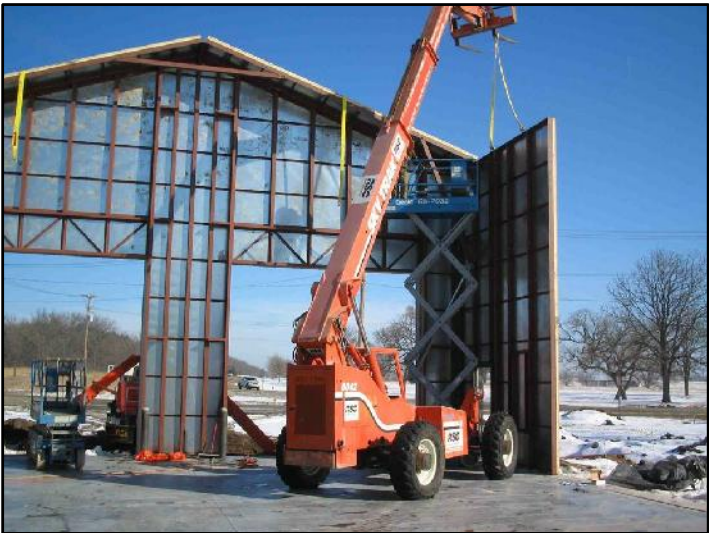
BOLT & ANCHOR BOTH SECTIONS INTO PLACE.
