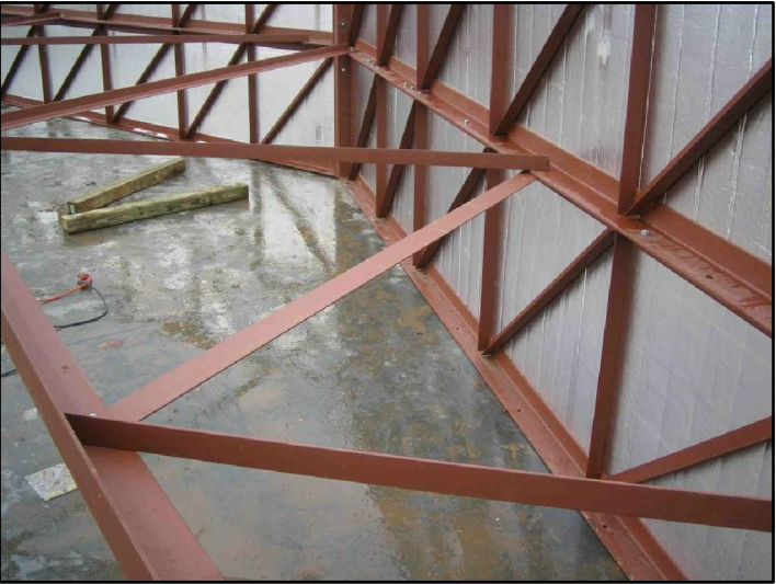
INSTALL THE EAVE ANGLES (4 TOTAL) & TRUSS & WEB MEMBERS TO THE ROOF SECTION.
