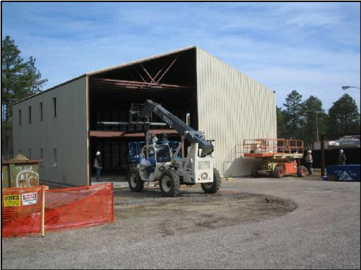
THE LAST END WALL WILL BE DONE IN HALF SECTIONS.
