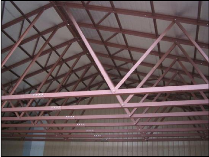
CONTINUE TO INSTALL THE INTERMEDIATE TRUSS WORK AFTER EVERY ROOF SECTION IS SET. AFTER ALL TRUSSES ARE IN PLACE, INSTALL THE BRIDGING ANGLES.
