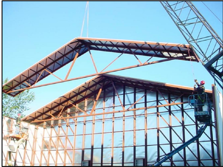
WHEN LIFTING ANY SECTION, A TAG LINE SHOULD BE USED.
