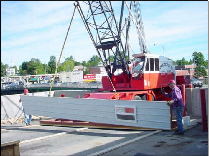
HEAVY PANELS OR PANELS WITH UNEVEN WEIGHT MAY REQUIRE TWO (2) PICKING POINTS.
