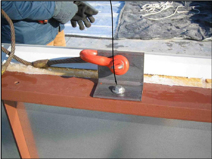
BOLT THE KELLY SUPPLIED LIFTING ANGLE TO THE PANEL TO LIFT OUT OF THE RACK AND MOVE TO THE STAGING AREA.
