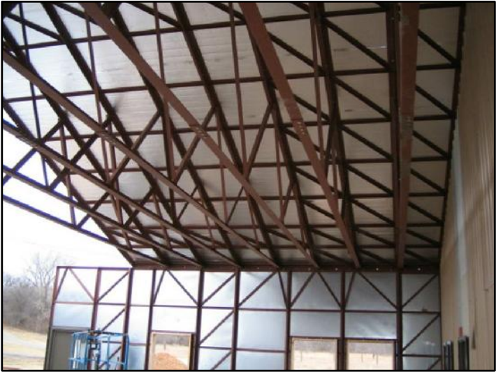
CONTINUE SETTING WALL SECTIONS & ROOF SECTIONS THROUGHOUT THE FULL LENGTH OF THE BUILDING.
