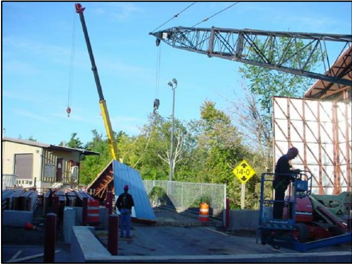
INSTALL THE EAVE ANGLES (4 TOTAL) & TRUSS & WEB MEMBERS TO THE ROOF SECTION.
