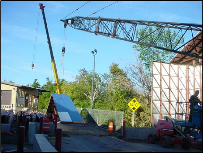
RIG TO THE FACTORY SUPPLIED PICKING FIXTURE IN THE RIDGE ANGLES & BEGIN TO ROLL THE ROOF SECTION OVER.
