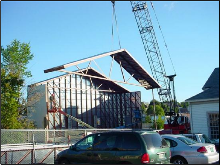
MAKE SURE THE OVERLAPPING EDGE IS TOWARDS THE ALREADY ASSEMBLED BUILDING SECTION.
