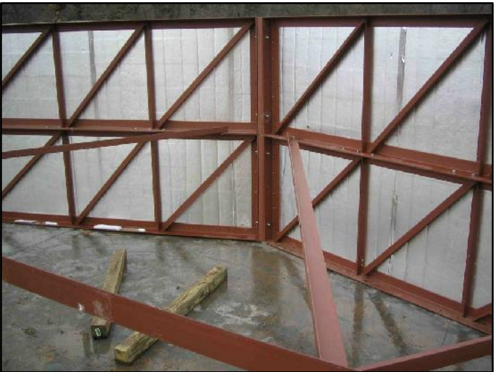
BUILD A 6'-0" ROOF SECTION ON ITS SIDE.
