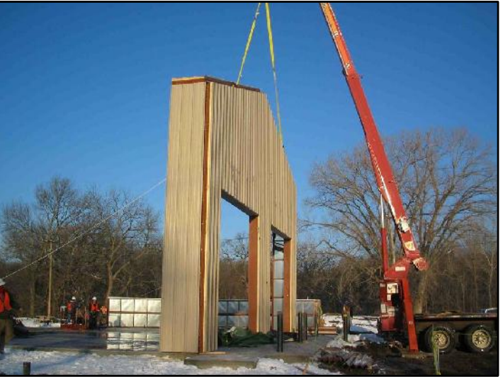
REMOVE TIPPING FEET BEFORE SETTING INTO PLACE.
