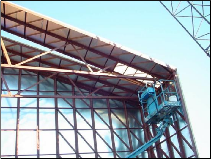
MAKE SURE THE ROOF SHEETING HAS OVERLAPPED THE ALREADY ASSEMBLED ROOF & BEGIN BOLTING AT THE EAVE.
