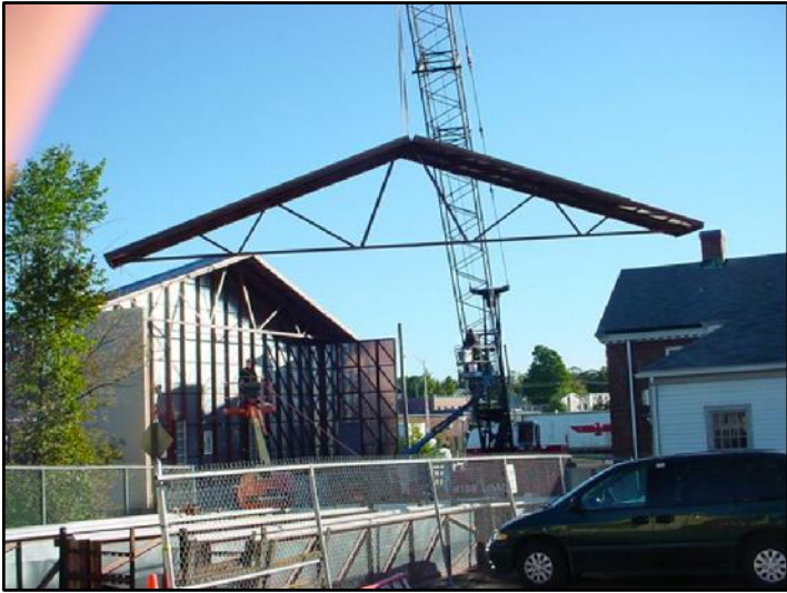
CRANE ROOF SECTIONS SLOWLY TOWARD THE BUILDING.
