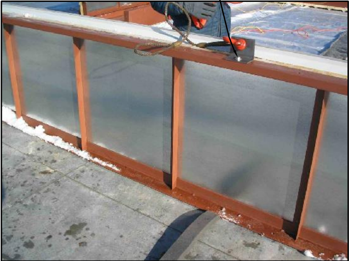
MAKE SURE THE LIFTING ANGLE IS CENTERED ON THE PANEL.
