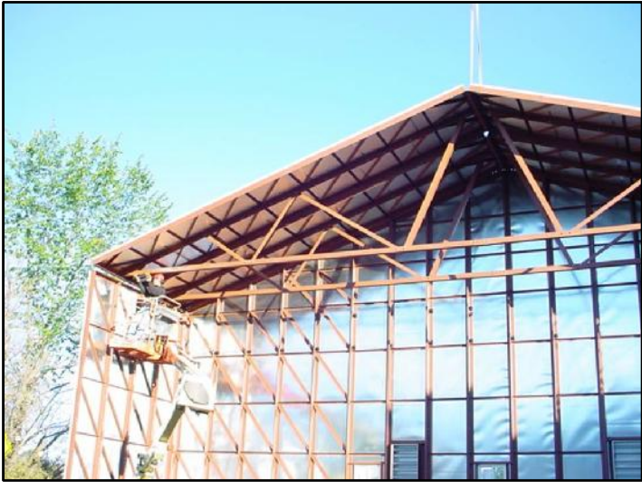
CONNECT THE OTHER EAVE & WORK YOUR WAY UP TO THE RIDGE.
