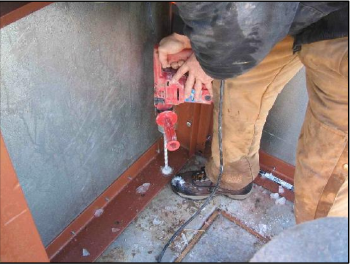
LINE UP THE INSIDE OF THE PANEL WITH THE CHALK LINE, SQUARE UP THE CORNERS, & INSTALL THE CONCRETE ANCHORS. SEE ANCHORING DETAILS FOR ANCHOR HOLE LOCATIONS.
