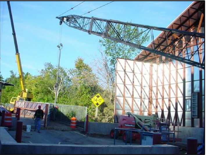
RIG TO THE FACTORY SUPPLIED PICKING FIXTURE IN THE RIDGE ANGLES & BEGIN TO ROLL THE ROOF SECTION OVER.
