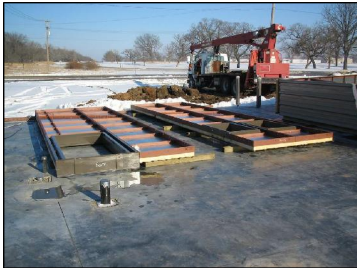
BEGIN BUILDING THE FIRST END WALL ON THE GROUND WITH THE EXTERIOR SHEETING DOWN. IT'S BEST TO BUILD THIS SECTION ON WOOD TO PREVENT SHEETING DAMAGE.
