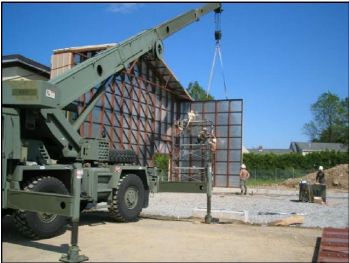
SUB-ASSEMBLE TWO (2) SIDE WALL SECTIONS (ONE EACH SIDE) ON THE GROUND AND LIFT INTO PLACE. DO THIS IN 12'-0" SECTIONS.
