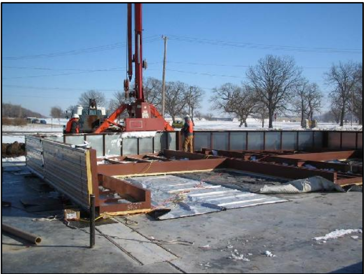
CONNECT THE FIRST ROOF & WALL PANELS TO THE CORNER & GABLE ERECTION ANGLES. ATTACH LARGE LIFTING ANGLES WITH 5/8" BOLTS & NUTS. NOTE: PANEL LAPS SHOULD BE DOWN TOWARD THE GROUND.
