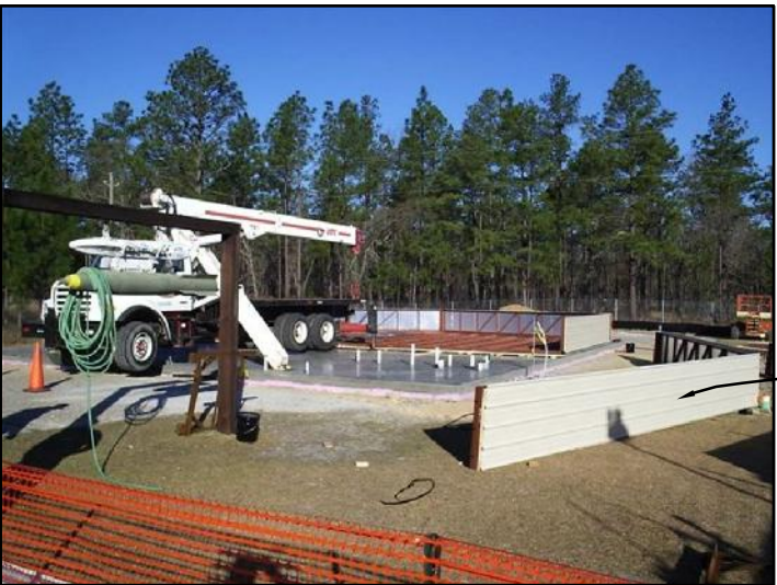
BEFORE LIFTING THE END WALL, TEMPORARILY ATTACH THE FIRST TRUSS FOR BRACING DURING LIFT, SNAP A CHALK LINE ON THE BUILDING SLAB, & TEMPORARILY ATTACH TIPPING FEET.
