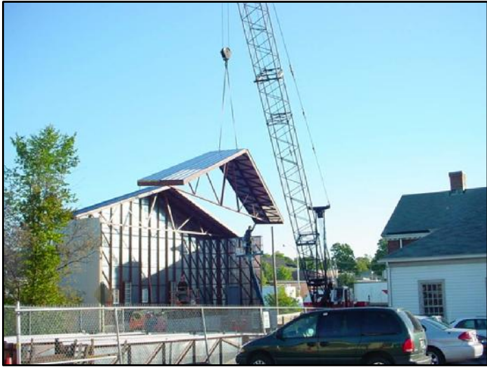
WORKERS SHOULD BE READY TO RECEIVE THE ROOF SECTION & BEGIN ALIGNING HOLES.
