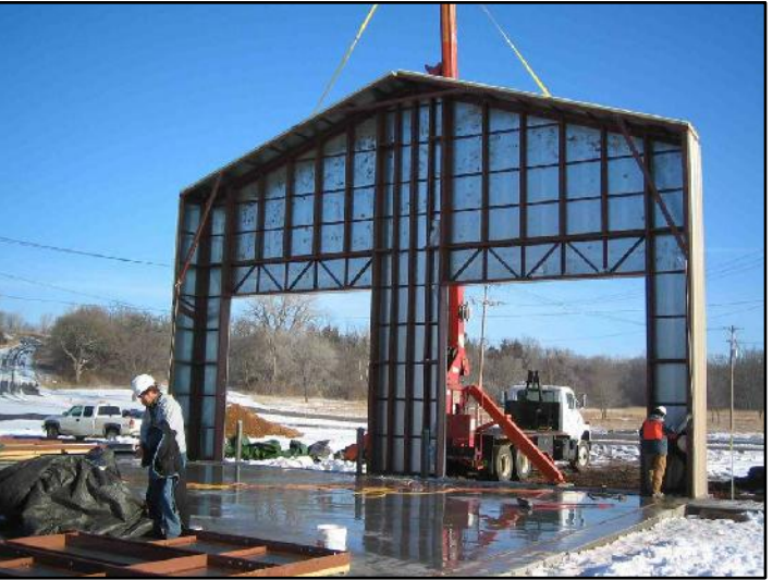
COMPLETED END WALL, SET & READY FOR WALLS & ROOF SECTIONS.
