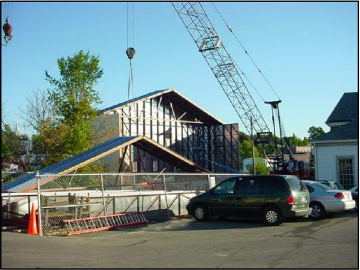
SUB-ASSEMBLED 6'-0" ROOF SECTION READY TO BE LIFTED INTO PLACE.
