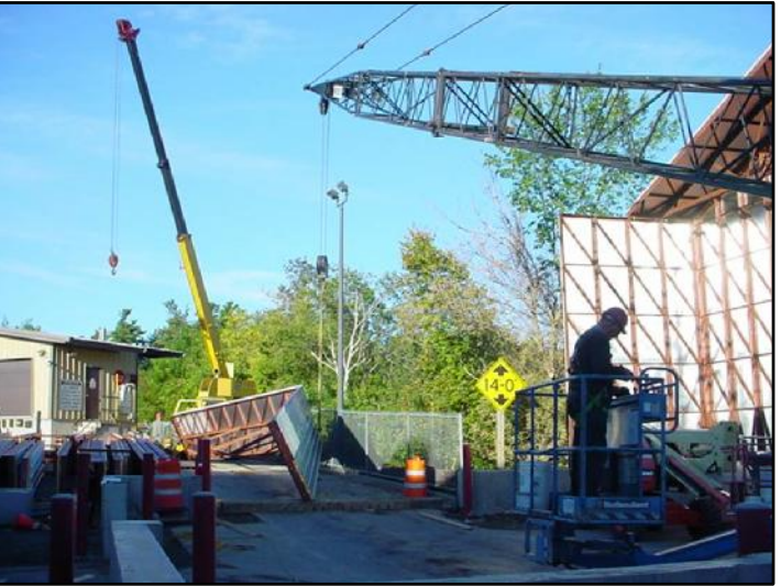
SLOWLY & SAFELY ROLL THE ROOF SECTION UP.
