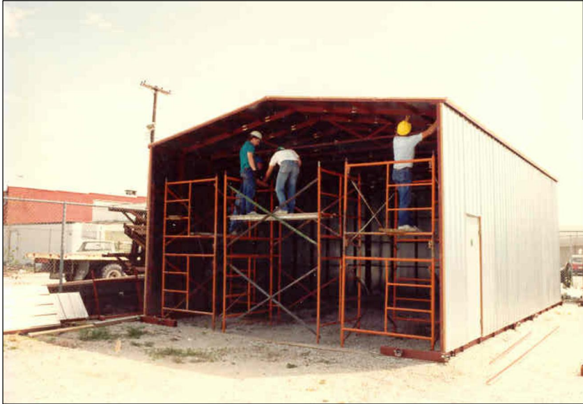
STEP #9 CONTINUE INSTALLING SIDEWALL & ROOF PANELS FOR THE REMAINING LENGTH OF THE BUILDING.
