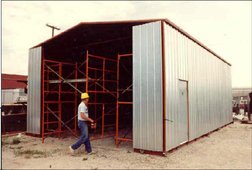
STEP #10 START ATTACHING THE FINAL END WALL PANELS (RIGHT TO LEFT) TO THE PREVIOUS SECTION OF BUILDING. CONTINUE ATTACHING WALL PANELS UNTIL ENTIRE END WALL HAS BEEN ATTACHED.
