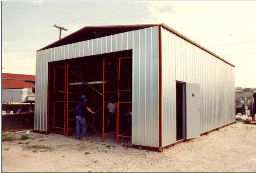
STEP #11 AFTER END WALL HAS BEEN ATTACHED, ATTACH THE GABLE CLOSURE PANELS TO THE PREVIOUS SECTION OF BUILDING. (NOTE: YOU WILL NEED PEOPLE ON THE OUTSIDE OF THE BUILDING LIFTING OR GUIDING THE PANELS INTO PLACE AND PEOPLE ON THE INSIDE ATTACHING THE PANELS TO THE BUILDING.)
