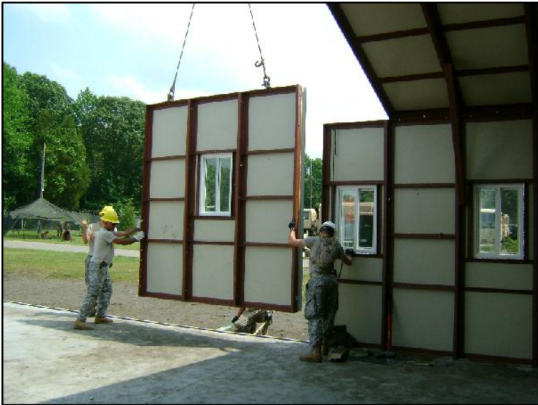
STEP #15: LIFT TWO (2) SIDEWALL SECTIONS INTO PLACE (ONE ON EACH SIDE) USING A CRANE & SLINGS. LOWER THE SECTIONS INTO THE CORRECT LOCATION USING THE CHALK LINE. BOLT THE SECTIONS TO THE REST OF THE BUILDING AND ANCHOR THEM DOWN. DO NOT FORGET THE BASE SEAL UNDER THE WALL PANELS.
