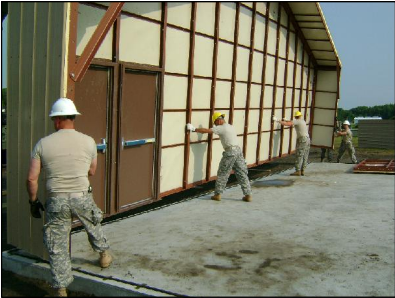
STEP #13: SET THE ENDWALL SECTION INTO THE CORRECT LOCATION USING A CHALK LINE LAYOUT. REFER TO THE FOUNDATION PREPARATION PLAN FOR THE CHALK LINE LOCATIONS. BE SURE TO PUT THE BASE SEAL UNDER THE PANELS AND REMOVE THE END WALL TIPPING FEET BEFORE SETTING THE ENDWALL SECTION DOWN.
