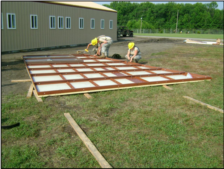
STEP #18: SUB-ASSEMBLE THE FINAL ENDWALL IN HALVES OR THIRDS (DEPENDING ON THE BUILDING SIZE) ON THE GROUND AND LIFT INTO PLACE USING A CRANE AND SLINGS. SET THE PANELS ON WOOD DUNNAGE TO PROTECT THE SHEETING.
