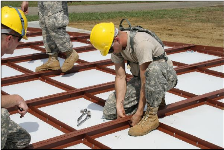
STEP #1: LAY OUT THE GABLE END PANELS MAKING SURE THAT THE SHEETING OVERLAPS ARE NESTING PROPERLY FROM ONE PANEL TO THE NEXT. GABLE PANELS ARE BOLTED TOGETHER USING 1/2" X 1 1/2" BOLTS AT APPROXIMATELY 3'-0" O.C. IT IS BEST TO LAY THE PANELS ON WOOD DUNNAGE TO PREVENT SHEETING DAMAGE.
