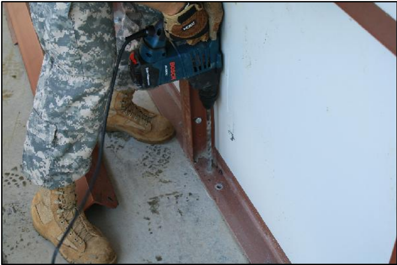
STEP #14: DRILL THE ANCHOR HOLES INTO THE CONCRETE USING A MASONRY DRILL. THE ANCHOR HOLES ARE FACTORY DRILLED IN THE BOTTOM OF THE WALL PANELS. ANCHOR THE ENDWALL SECTION DOWN AND REMOVE THE TEMPORARY KNEE & RIDGE BRACES.
