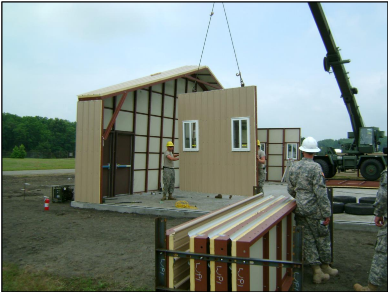
STEP #15: LIFT TWO (2) SIDEWALL SECTIONS INTO PLACE (ONE ON EACH SIDE) USING A CRANE & SLINGS. LOWER THE SECTIONS INTO THE CORRECT LOCATION USING THE CHALK LINE. BOLT THE SECTIONS TO THE REST OF THE BUILDING AND ANCHOR THEM DOWN. DO NOT FORGET THE BASE SEAL UNDER THE WALL PANELS.
