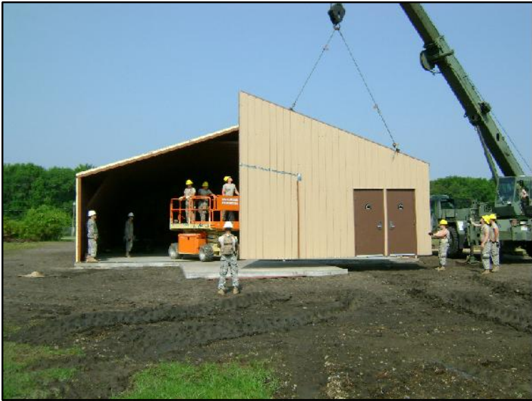
STEP #18: SUB-ASSEMBLE THE FINAL ENDWALL IN HALVES OR THIRDS (DEPENDING ON THE BUILDING SIZE) ON THE GROUND AND LIFT INTO PLACE USING A CRANE AND SLINGS. SET THE PANELS ON WOOD DUNNAGE TO PROTECT THE SHEETING.
