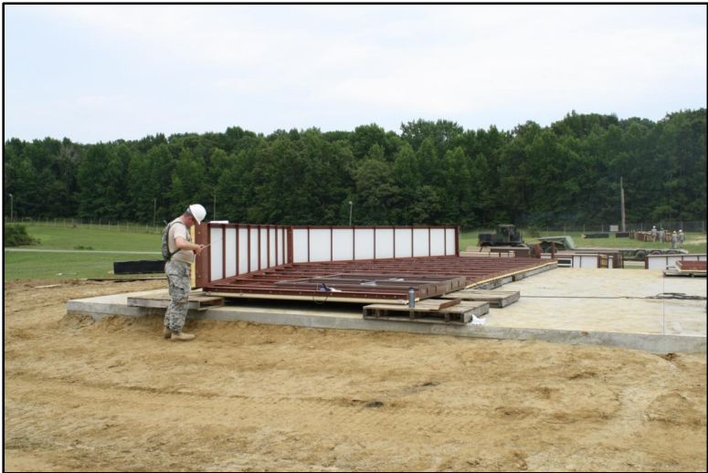
STEP #3: ATTACH THE FIRST 3'-0" OF ROOF PANELS TO THE SUB-ASSEMBLED ENDWALL PANELS BY CONNECTING THE ROOF PANELS TO THE FLAT LEG OF THE 90° GABLE ERECTION ANGLE. IT IS VERY IMPORTANT TO NOTE THAT THE OVERLAP ON THE ROOF PANELS MUST FACE DOWN OR TOWARDS THE STARTING END OF THE BUILDING. MAKE SURE THE EAVE & RIDGE ANGLES ARE ATTACHED TO THE ROOF PANELS BEFORE INSTALLING ANY SIDEWALL PANELS.
