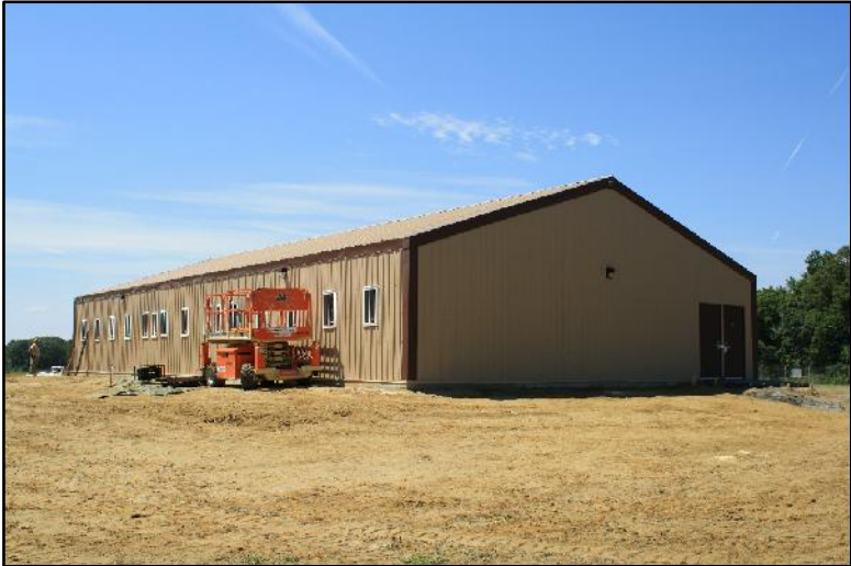
STEP #20: AFTER ALL PANELS AND KNEE/RIDGE BRACES ARE IN PLACE, ALL FLASHING AND OTHER COMPONENTS CAN BE INSTALLED.
