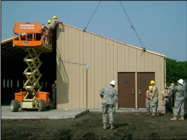
STEP #19: CONNECT THE ENDWALL SECTIONS TO THE REST OF THE BUILDING USING THE CORNER & GABLE ERECTION ANGLES.
