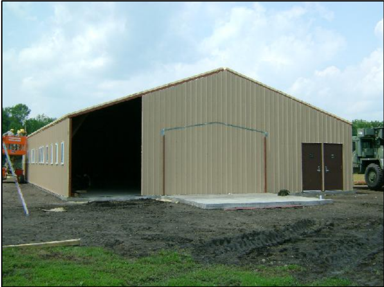
STEP #19: CONNECT THE ENDWALL SECTIONS TO THE REST OF THE BUILDING USING THE CORNER & GABLE ERECTION ANGLES.
