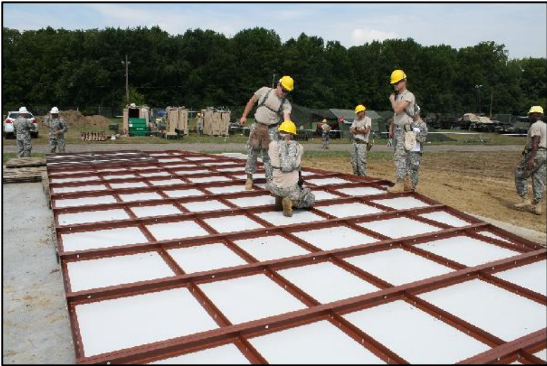
STEP #1: LAY OUT THE GABLE END PANELS MAKING SURE THAT THE SHEETING OVERLAPS ARE NESTING PROPERLY FROM ONE PANEL TO THE NEXT. GABLE PANELS ARE BOLTED TOGETHER USING 1/2" X 1 1/2" BOLTS AT APPROXIMATELY 3'-0" O.C. IT IS BEST TO LAY THE PANELS ON WOOD DUNNAGE TO PREVENT SHEETING DAMAGE.
