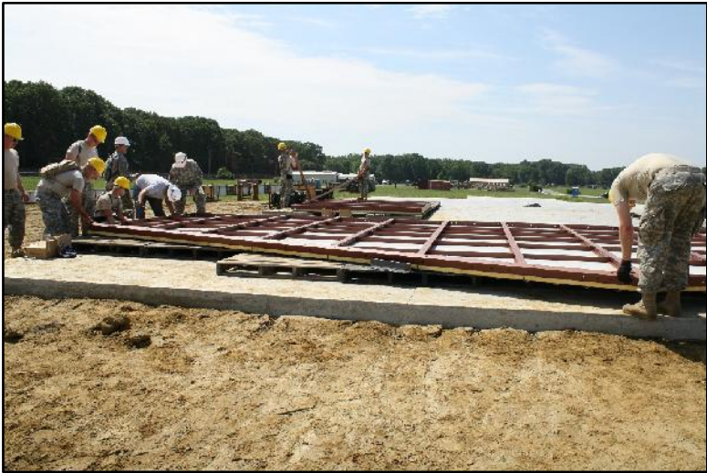
STEP #2: ATTACH THE 90° CORNER AND GABLE ERECTION ANGLES TO THE SUB-ASSEMBLED ENDWALL.
