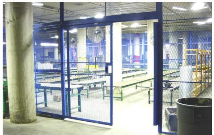
Expanded metal personnel doors are factory installed in a 4' x 8' panel that is interchangeable with other standard panels.
