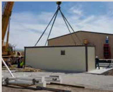
5. Drop in place
