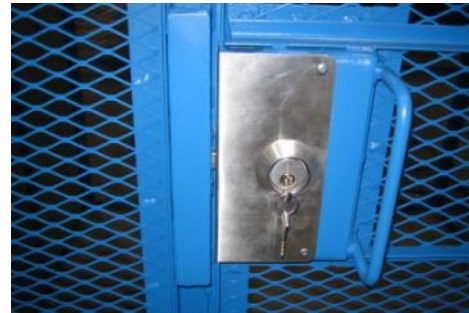
Doors Upgraded with Double Keyed Deadbolts for Higher Security
