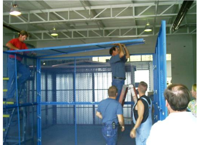
Roof Panels Placed onto Wall Panels
