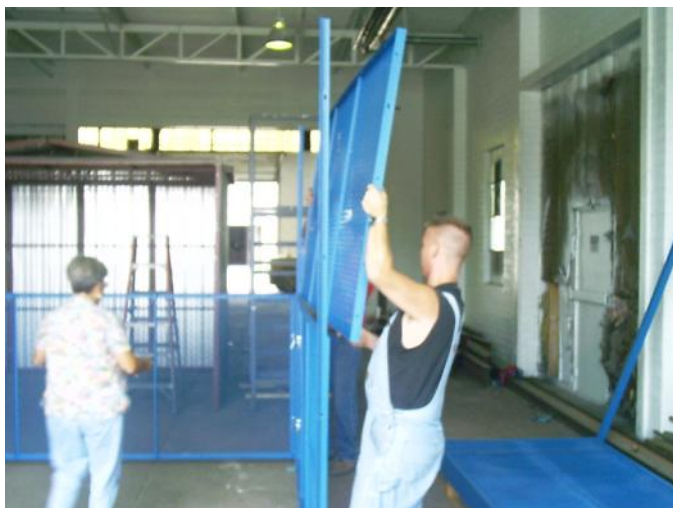
Upper Panels Stacked Onto Lower Panels
