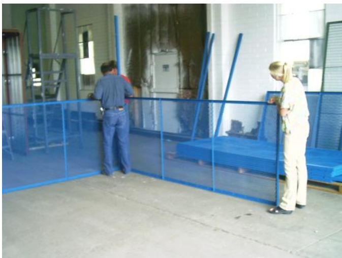
Lower Panels Moved Into Place By Hand
