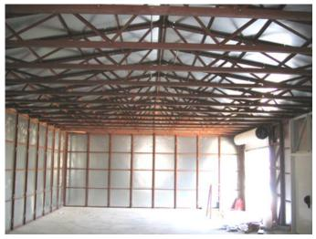
24' Wide Building Using Trussed Roof and Shear Walls
