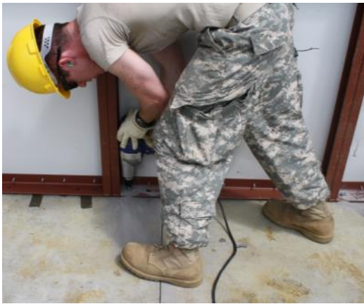
Concrete anchors are installed as the building is erected. No pre-set anchors required.
