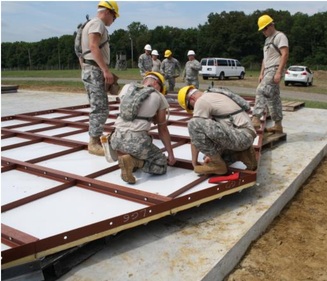
The first endwall is assembled on dunnage on the ground.
