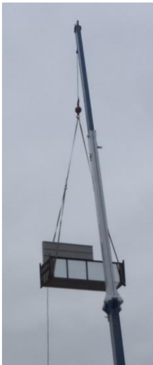
Panel Racks Being Moved with Slings by Overhead Crane
