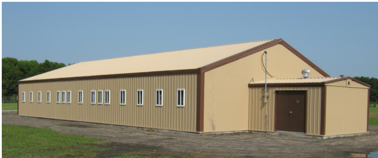
This 42' wide x 81' long classroom building was installed using troop labor without prior experience during a two week training deployment at Fort Dix in New Jersey.
