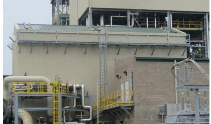
Steam Turbine Generator Building at Biofuel Power Plant in South Boston, VA
