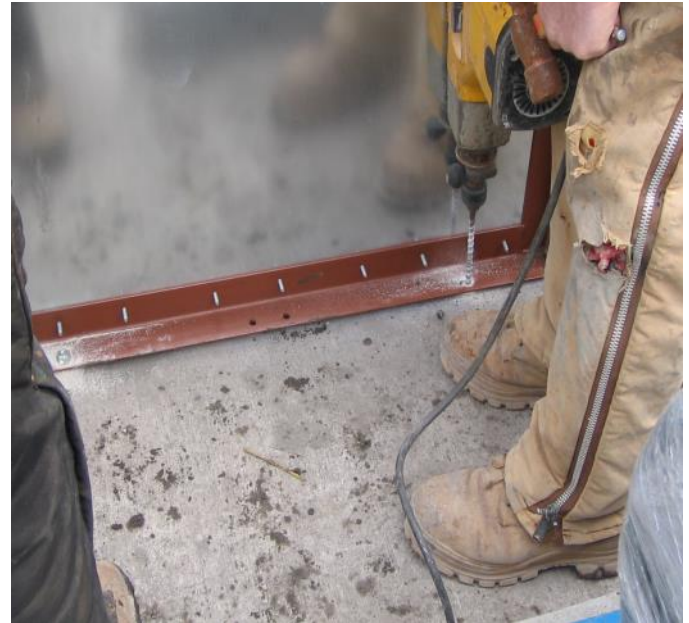
Drill Anchor Holes Through Panel Frames
