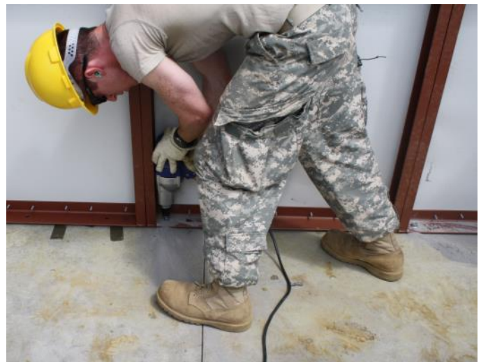
Install Anchor with Impact Wrench
