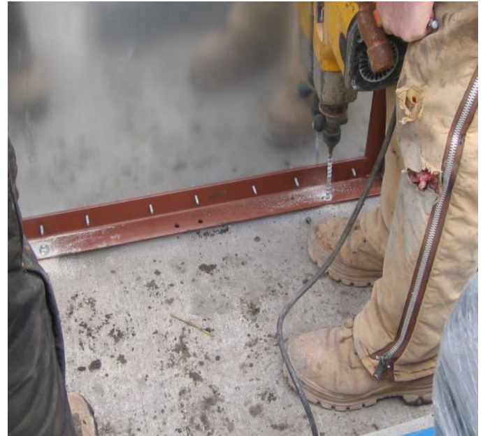
Drill Anchor Holes Through Panel Frames
