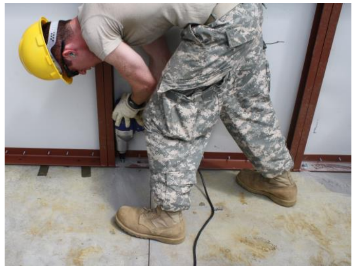
Install Anchor with Impact Wrench
