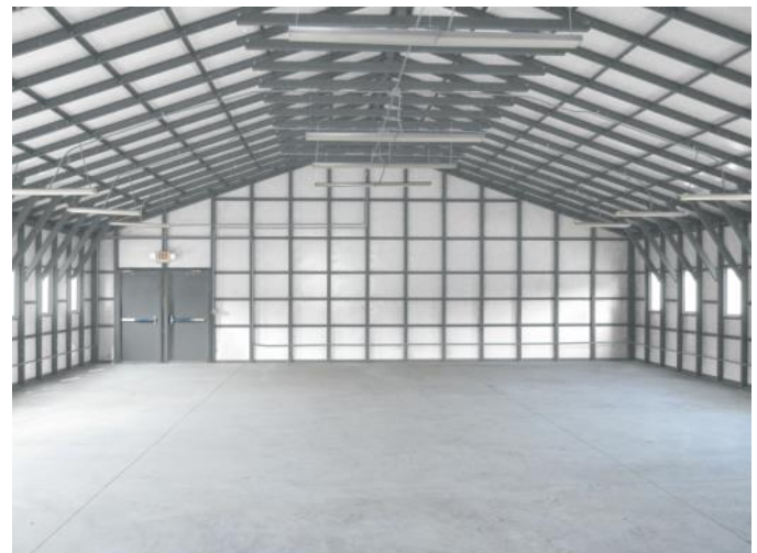
Painted Steel Liner
