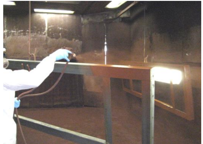
The Standard Red Primer Being Applied
