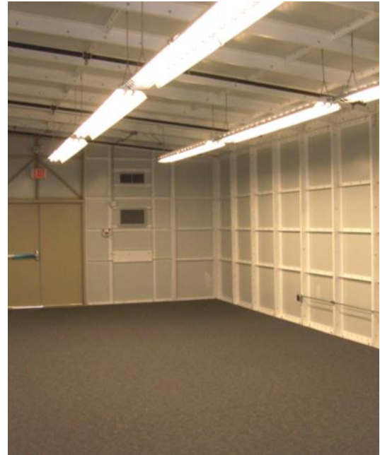
Painted Steel Liner
