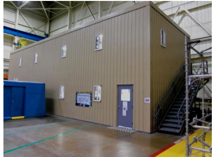
2-Story Flat Roof Interior Building used for Power Plant Outage Support
