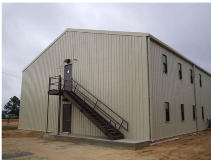
2-Story Administration Building at Ft. Bragg, NC
