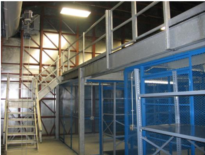
Building with Kelly Expanded Metal Lockers on First Floor and 2nd-Floor Storage Level
