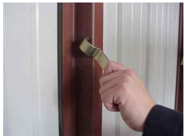
The Kelly Klosure "Locking Key" Can Be Used Where Possible In Lieu of Bolts in Temporary Use Structures For Faster Assembly and Disassembly
