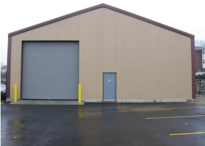
A 15’Wide Equipment Door in a Building’s Endwall
