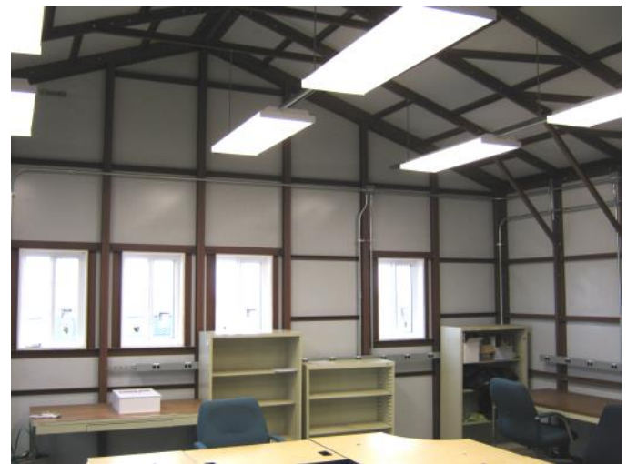
Building with Factory Installed Windows
