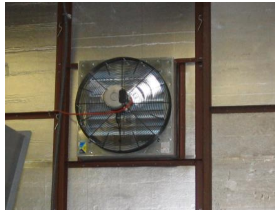
Wall Panel with Factory Installed Louver and Exhaust Fan
