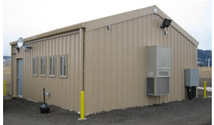
Building with Factory Installed Framing for Bard Wall-Mount HVAC Unit
