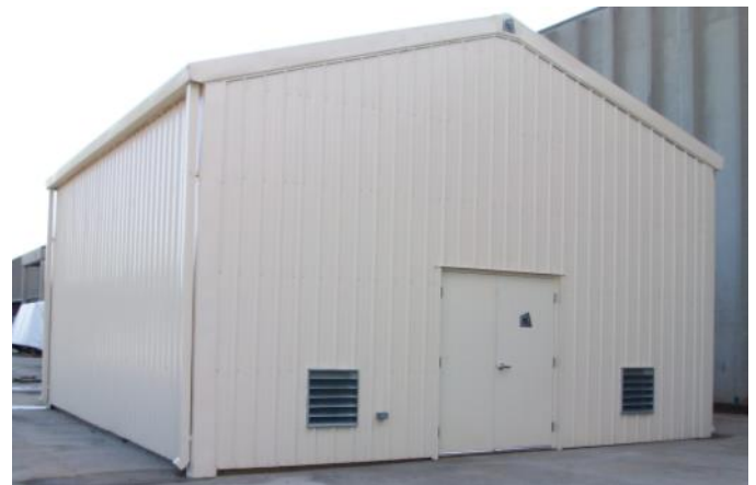
Building with Factory Installed Intake Louvers
