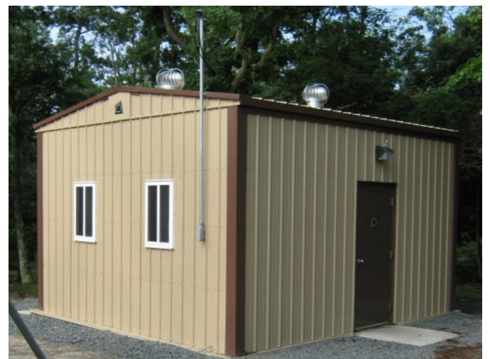
Building with Wind Driven Roof Ventilators
