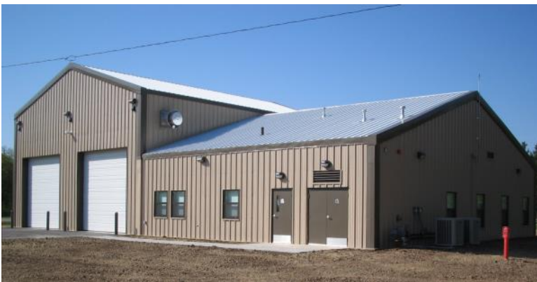
Fire Station at Fort Riley, KS with Anti-Terrorism Doors and Windows
