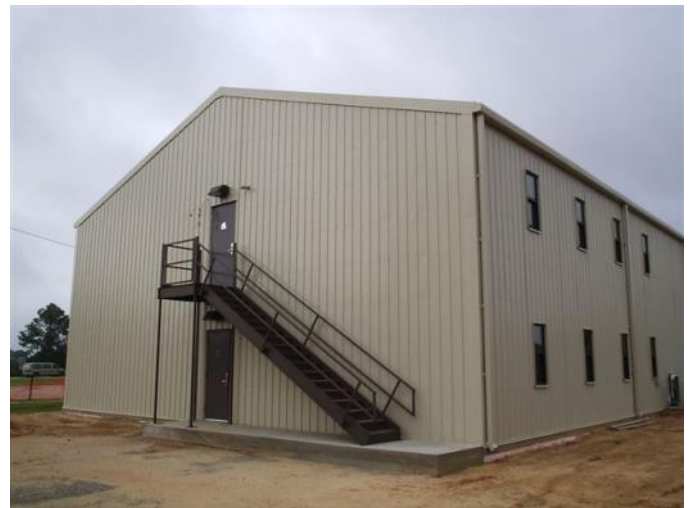
2-Story Kelly Klosure Relocatable Buildings at FT. Bragg, NC with Anti-Terrorism Doors and Windows used as Administration Buildings
